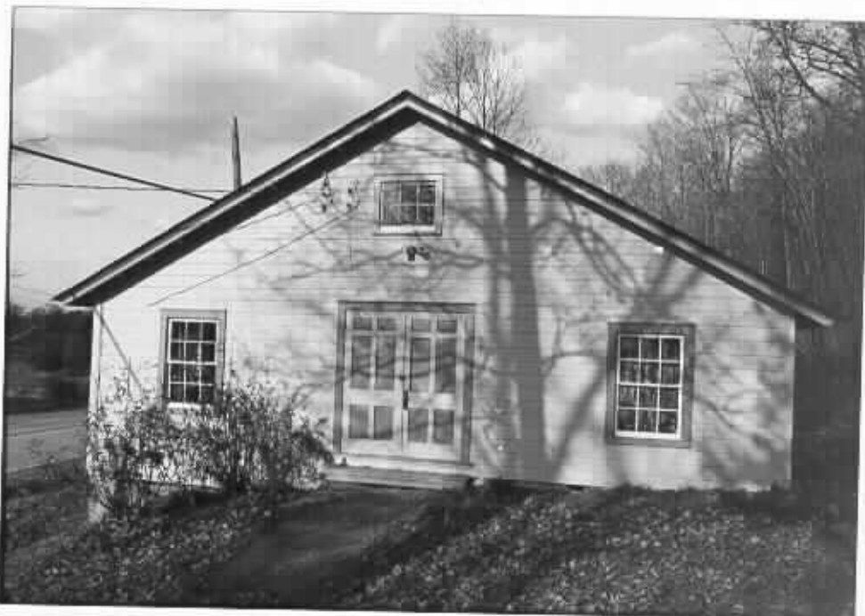
3. Parish hall, south facade
