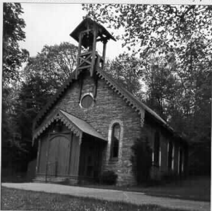
1. Front (west) and south elevations
