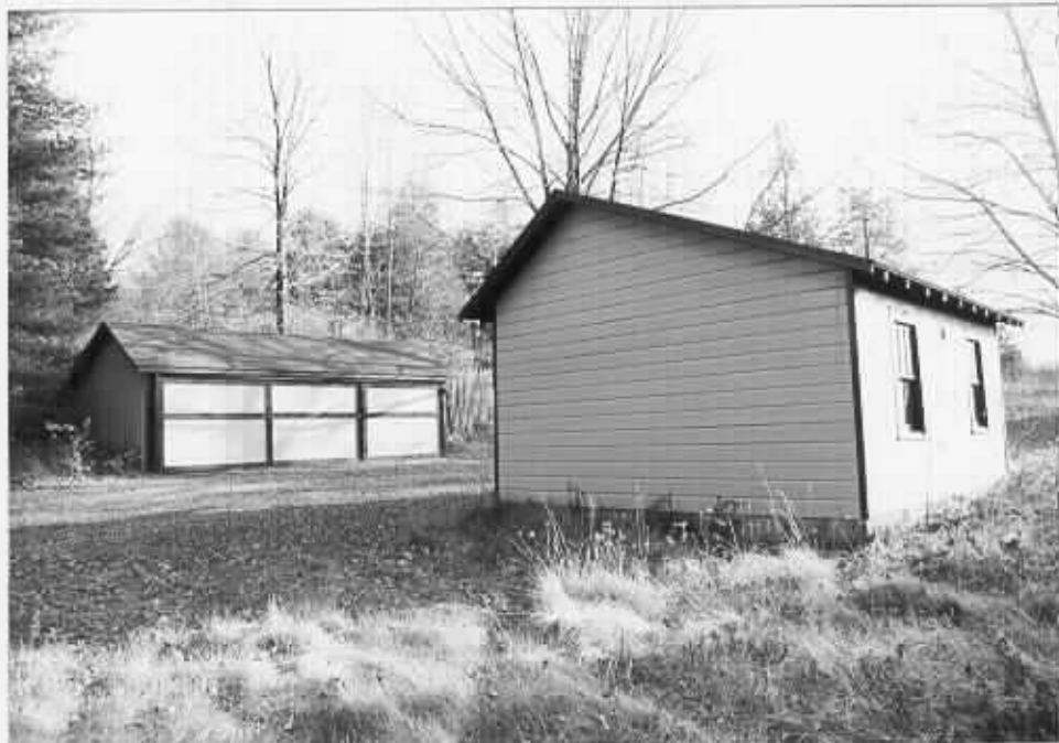
9. Sheds, north and west elevations
