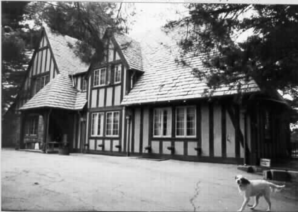
1. East facade, viewed from northeast
