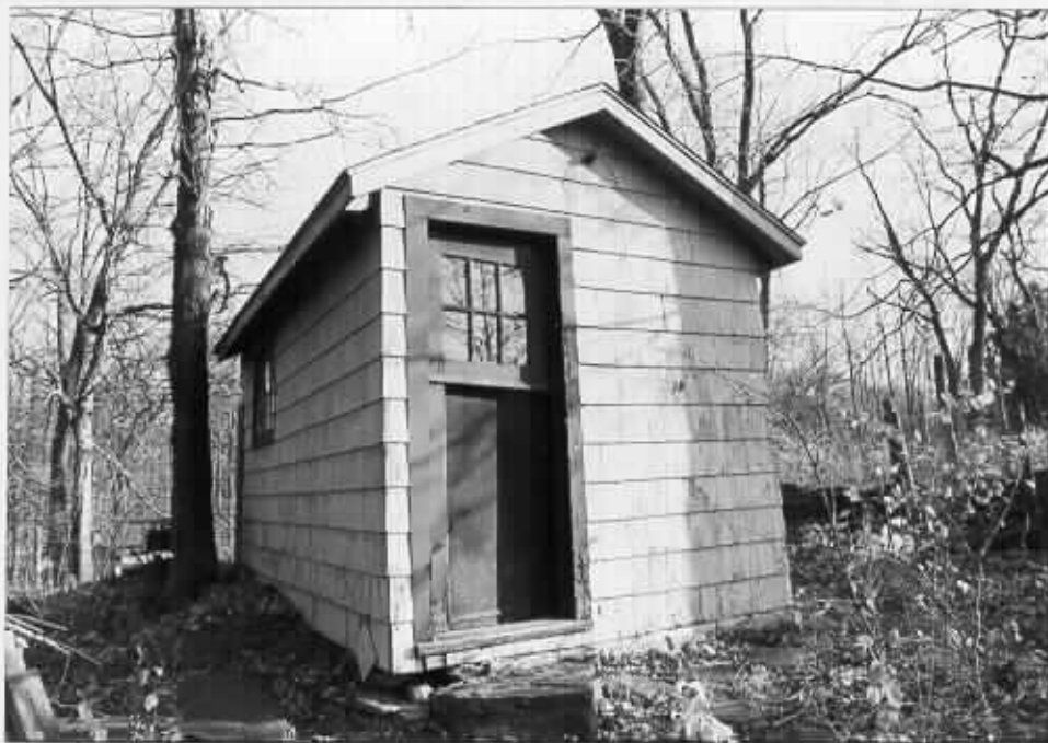
8. Shed, west facade and north elevation
